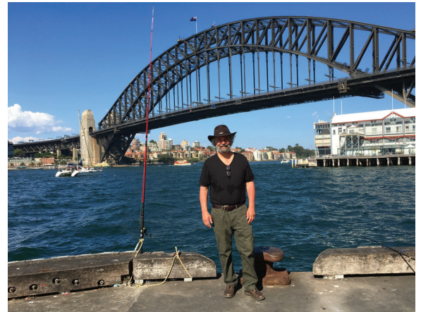
Sydney Harbour Bridge in Australia
